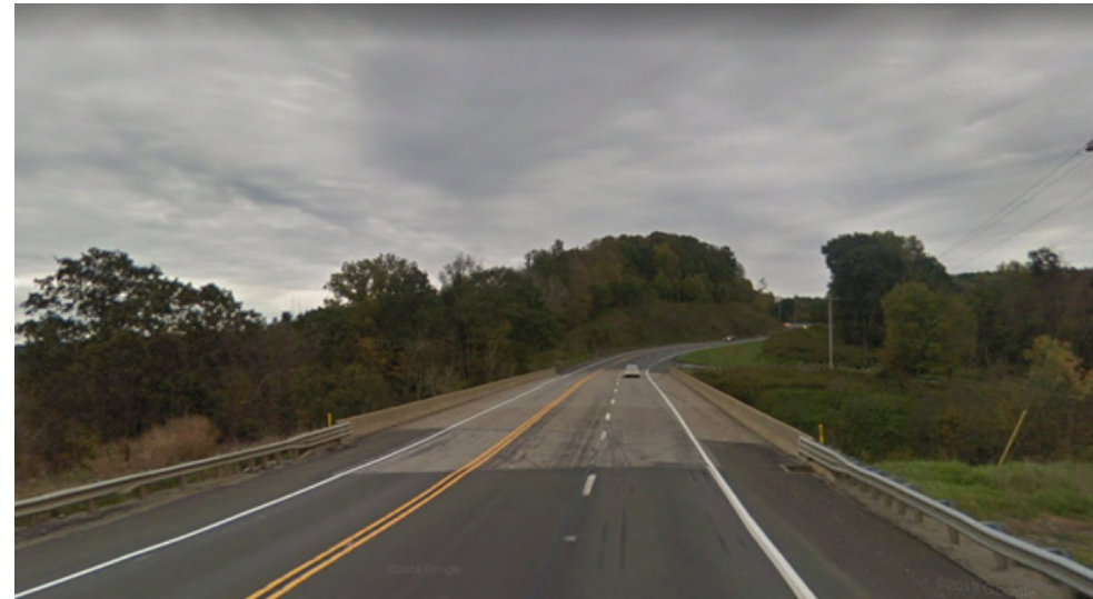
Colwell Cut Viaduct, Mahoning Township
