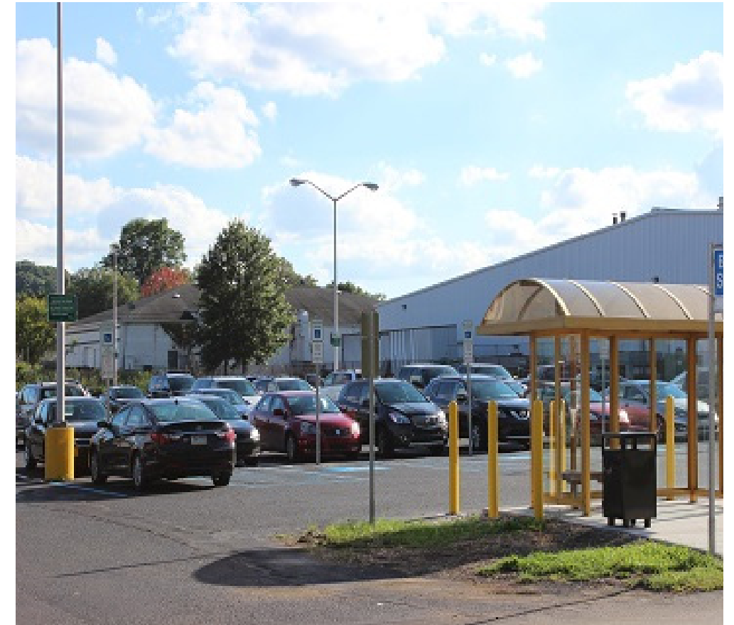
Harmar Park and Ride Facility
