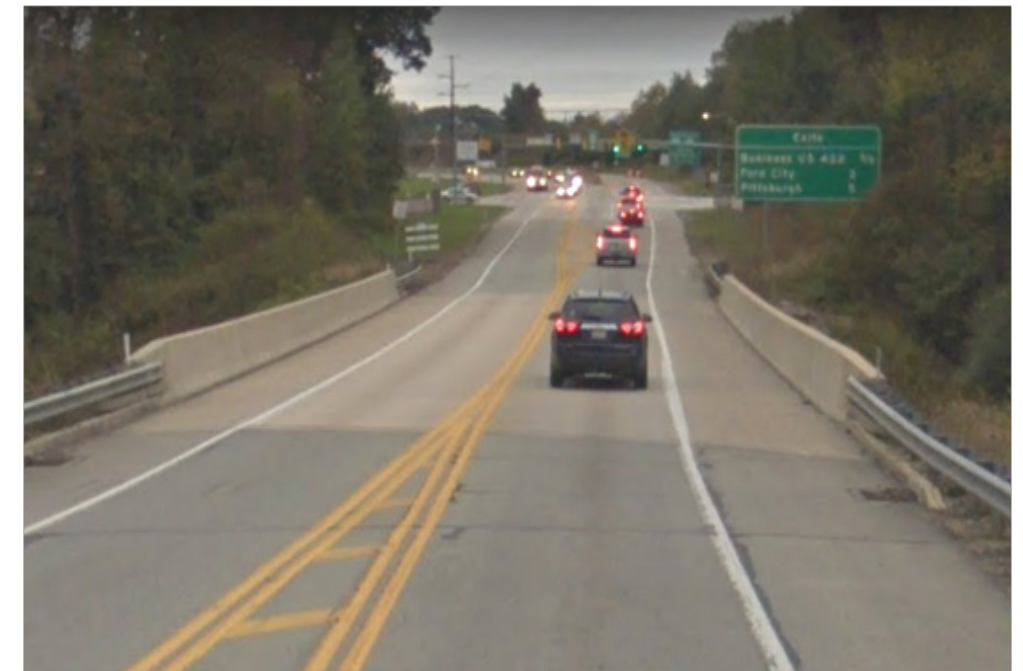
SR 28 Over Cowanshannock Creek
