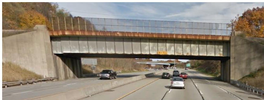
Figure 4-17: Railroad Overpass on SR 28 Northbound
