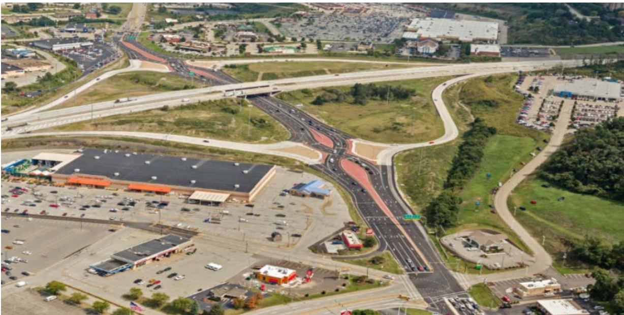
Figure 12: US 19/I-70 Diverging Diamond Interchange, South Strabane Township
